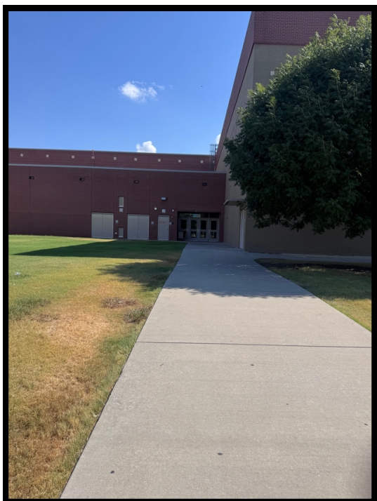
Prop Drop Off (Door 11)
